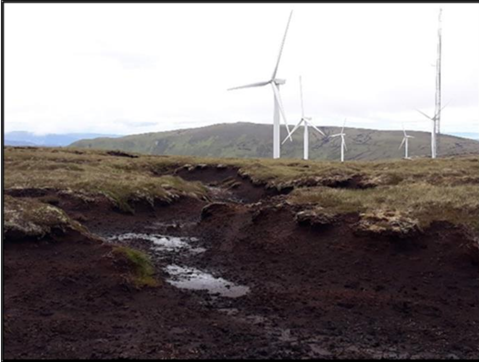
Plate 3: Before peatland restoration, note bare peat, vertical peat walls and eroded gully.
